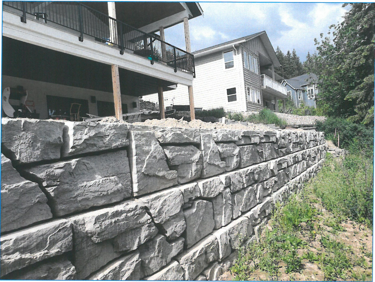
Figure 2 – Northern retaining wall (facing west)
