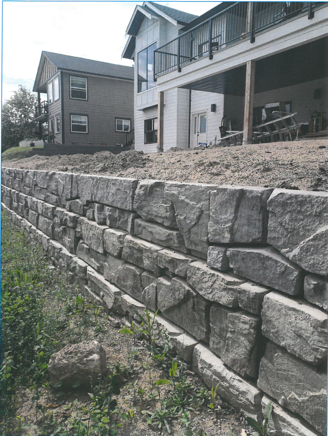
Figure 1 – Northern retaining wall (facing east)
