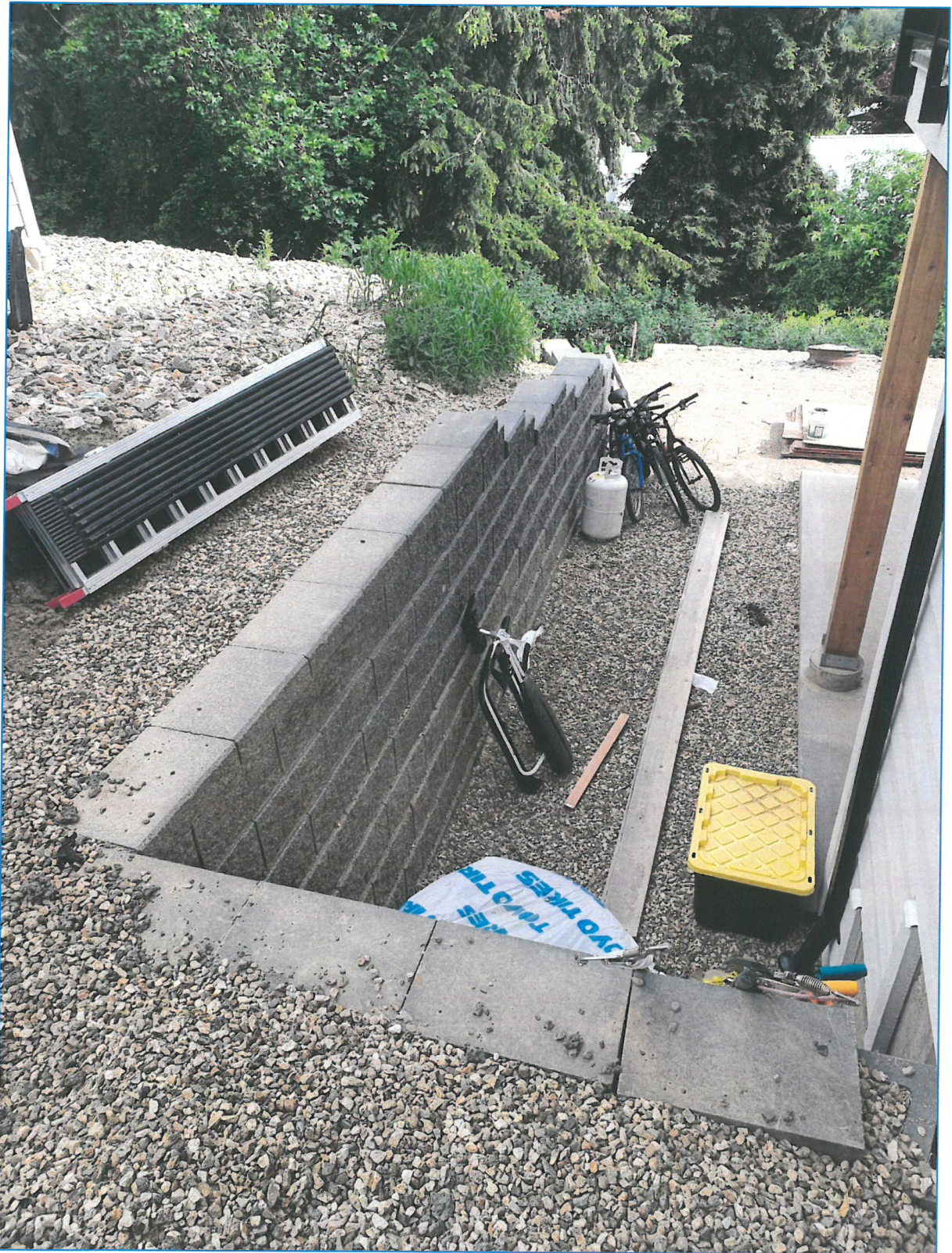
Figure 3 – Western retaining wall (facing south)
