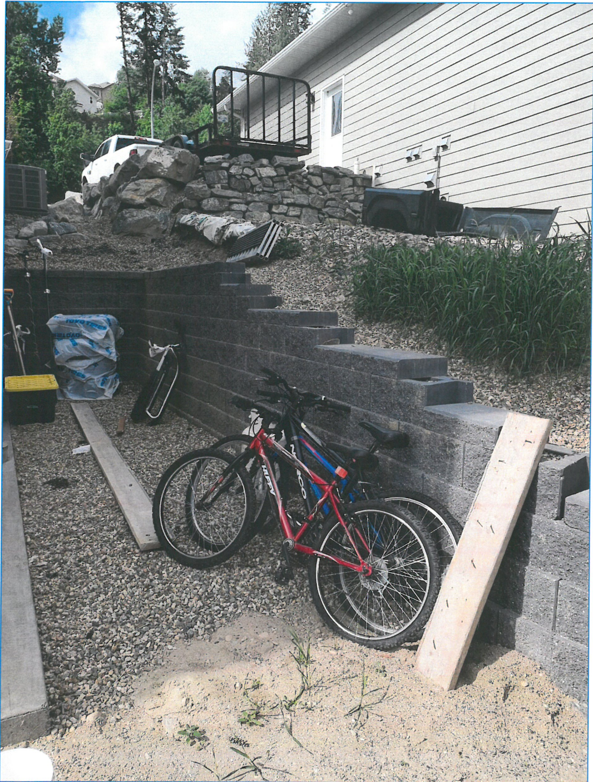
Figure 4 – Western retaining wall (facing south)
