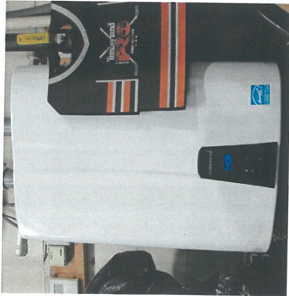
Photo #M3: Typical gas-fired domestic water heater.
