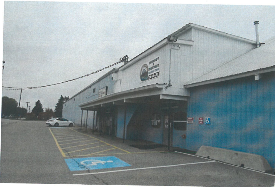
General view of the Site building
