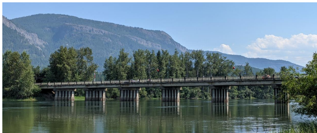
Figure AI-3: Highway 97A/Young Street Bridge on Shuswap River in Grindrod (2020)
