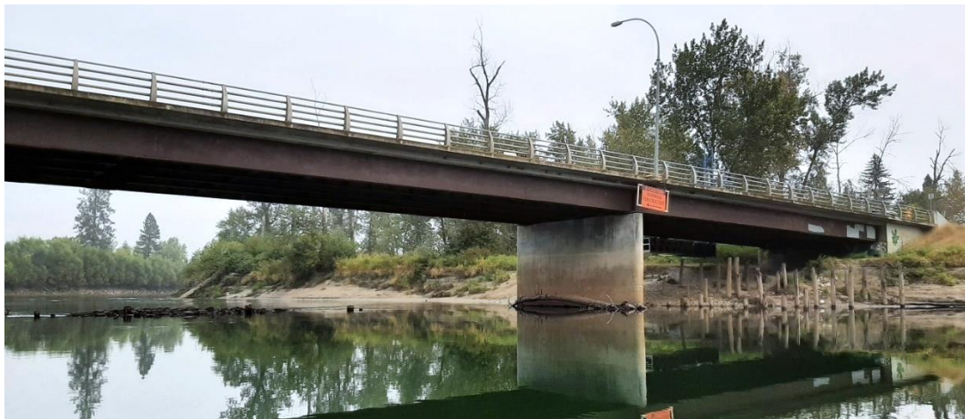
Figure AI-2: Bawtree Bridge on Shuswap River in Enderby (2020)
