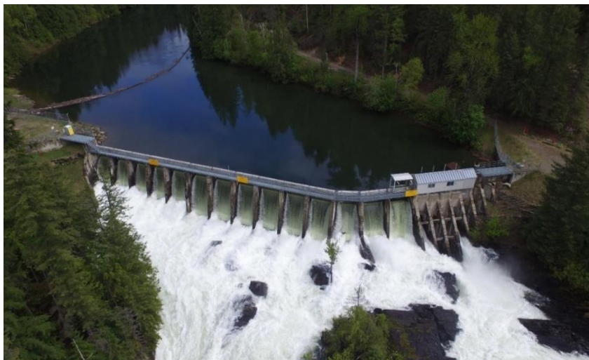
Note: Photograph taken on May 23, 2020. Flow over dam is approximately 180 m 3 /s.
