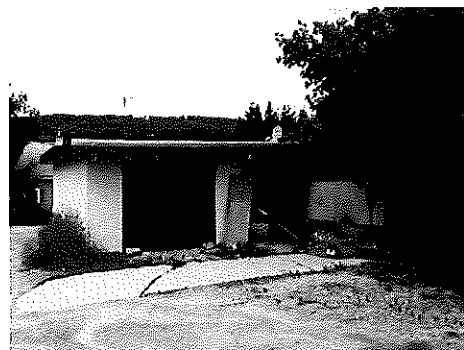
Photo 4: North elevation of attached garage
