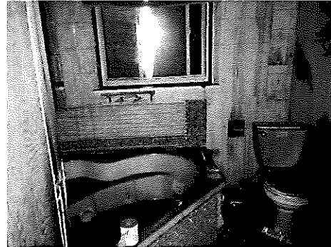
Photo 12: Main Level Bathroom
