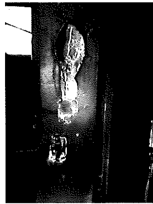
Photo 36: Damaged wall/missing cover
