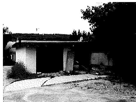
Photo 4: North elevation of attached garage
