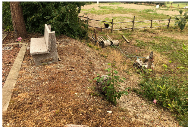
Figure 34: Existing Edge Condition, Source: LEES+Associates
