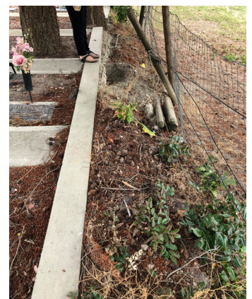
Figure 35: Existing Edge Condition, Source: LEES+Associates
