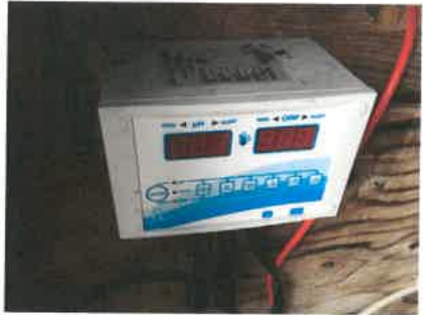
Figure 5 Chemical Feed System
