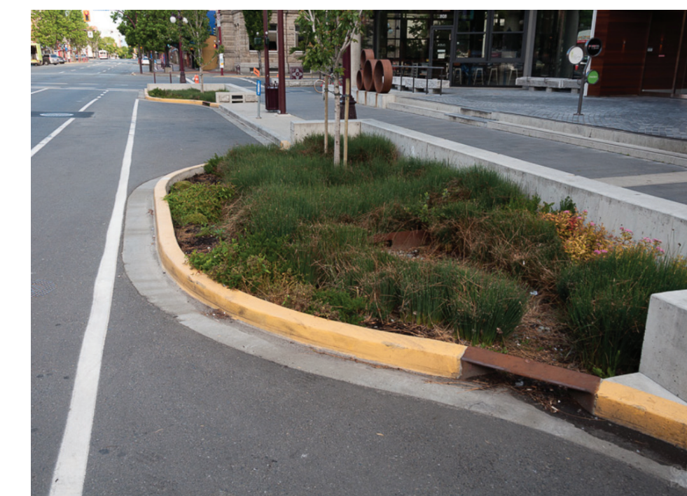
Curb break to allow water into rain garden
