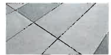
Cast-in-place concrete with sawcut joints
