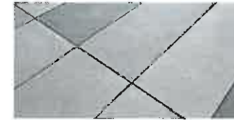
Cast in-place concrete with sawcut joints
