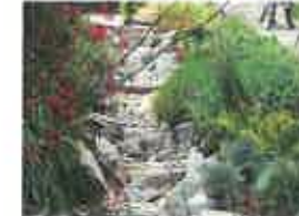
Stone infiltration bed and rain garden plantings
