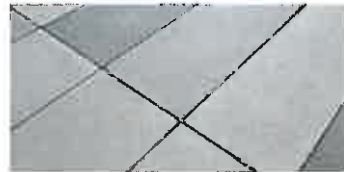
in place concrete
