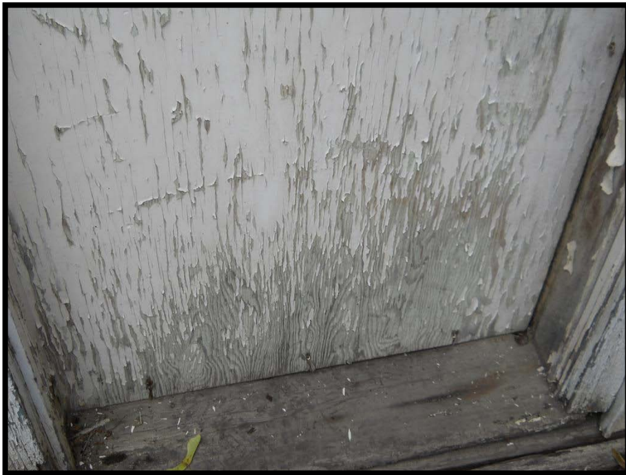
Photo 4: Lead-based white exterior/trim paint.
