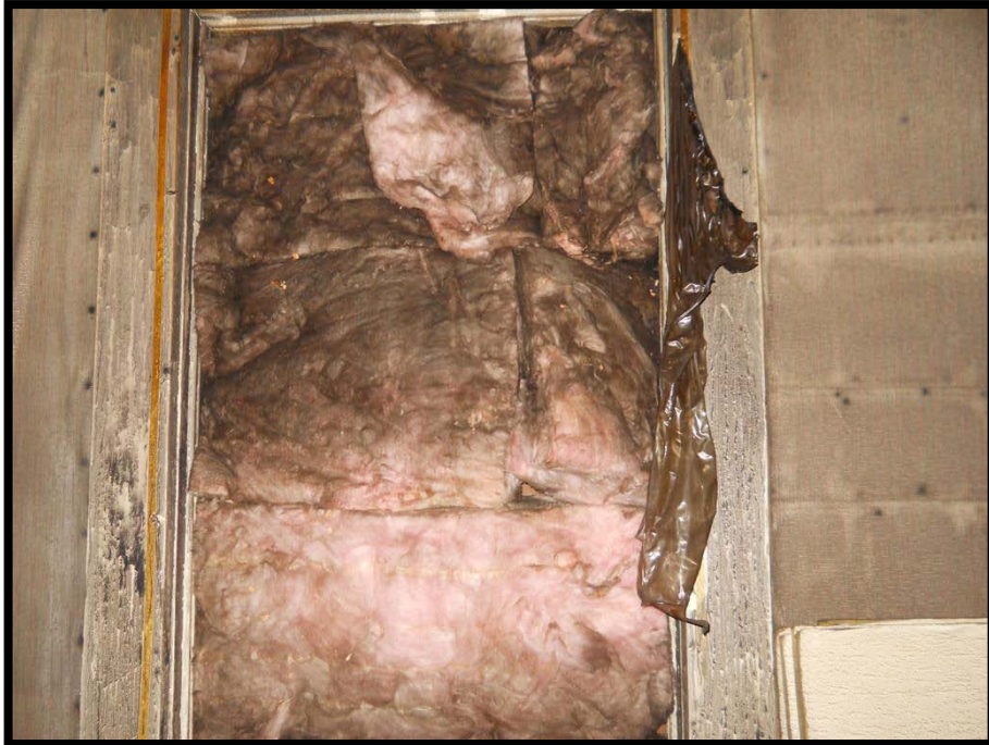
Photo 8: Visually non-asbestos fibreglass insulation.
