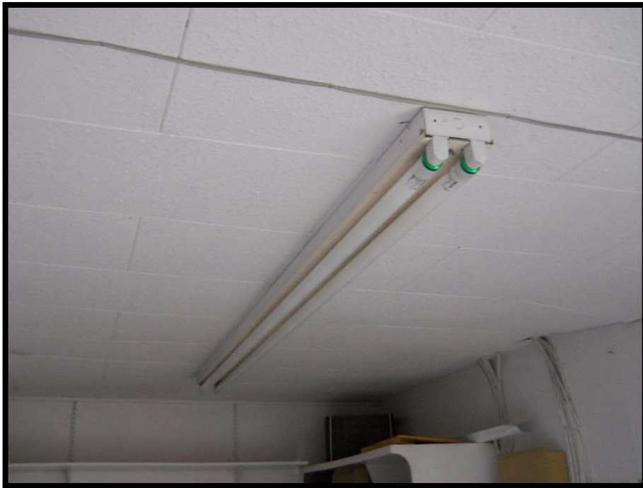
Photo 5: Light tubes contain mercury vapour and light ballasts contains PCBs.
