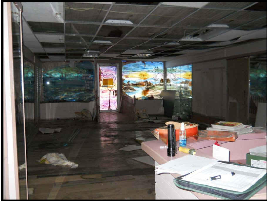
Photo 6: View of the main floor of the building.
