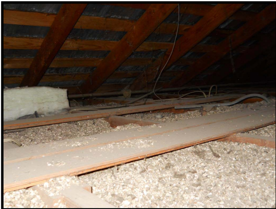
Photo 2: Asbestos-containing vermiculite insulation.
