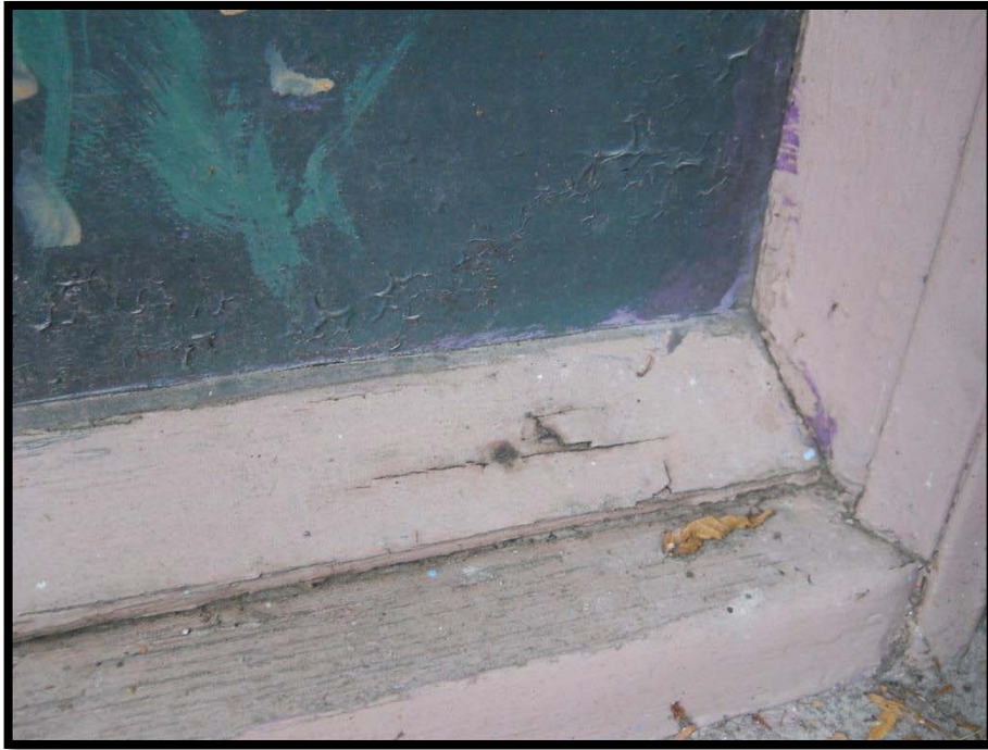
Photo 3: Lead-based brown exterior trim paint.
