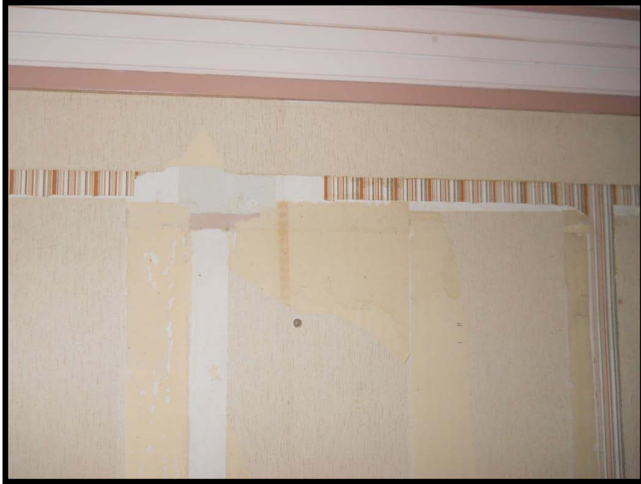
Photo 1: Drywall applied with asbestos-containing drywall joint compound.
