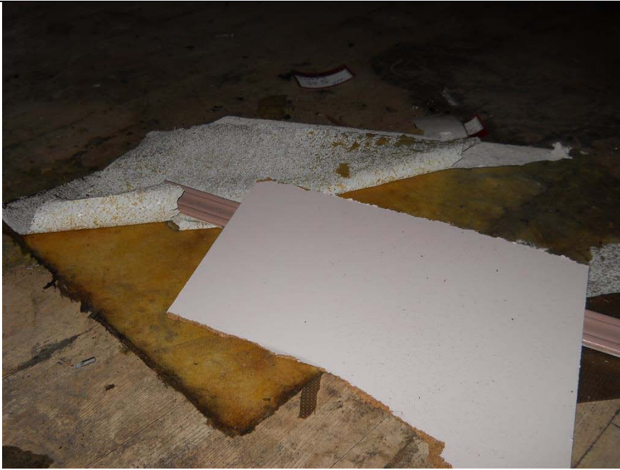
Photo 9: Visually non-asbestos fibreglass ceiling tile.
